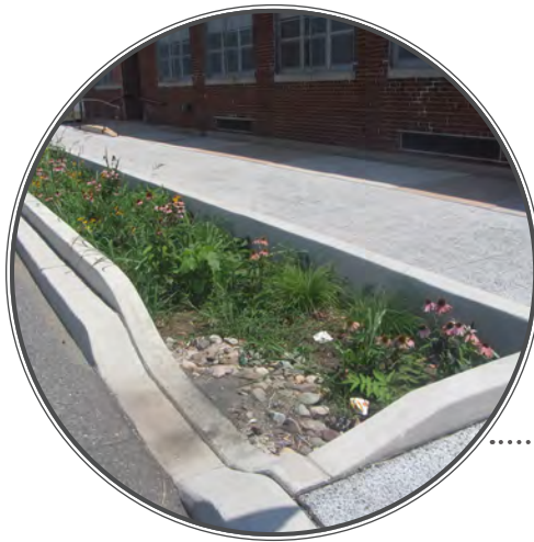
LOCATION: Camden, NJ This stormwater planter was designed to capture stormwater runoff from the street in front of the Brimm School in Camden, New Jersey.
